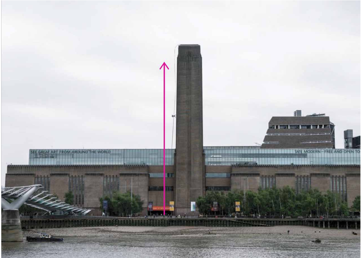
Fig.02. Proposed Location Path A: Tate Modern's chimney – east facing.
