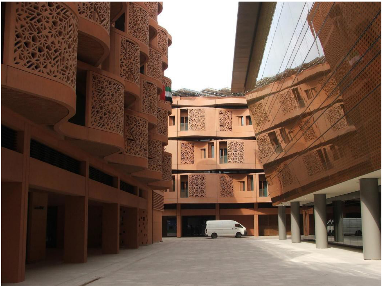
Figure 5 Terracotta façade of student dormitories designed by Foster & Partner, https://www.architecturalrecord.com/articles/7866-0-14-tower accessed May 1st 2026
