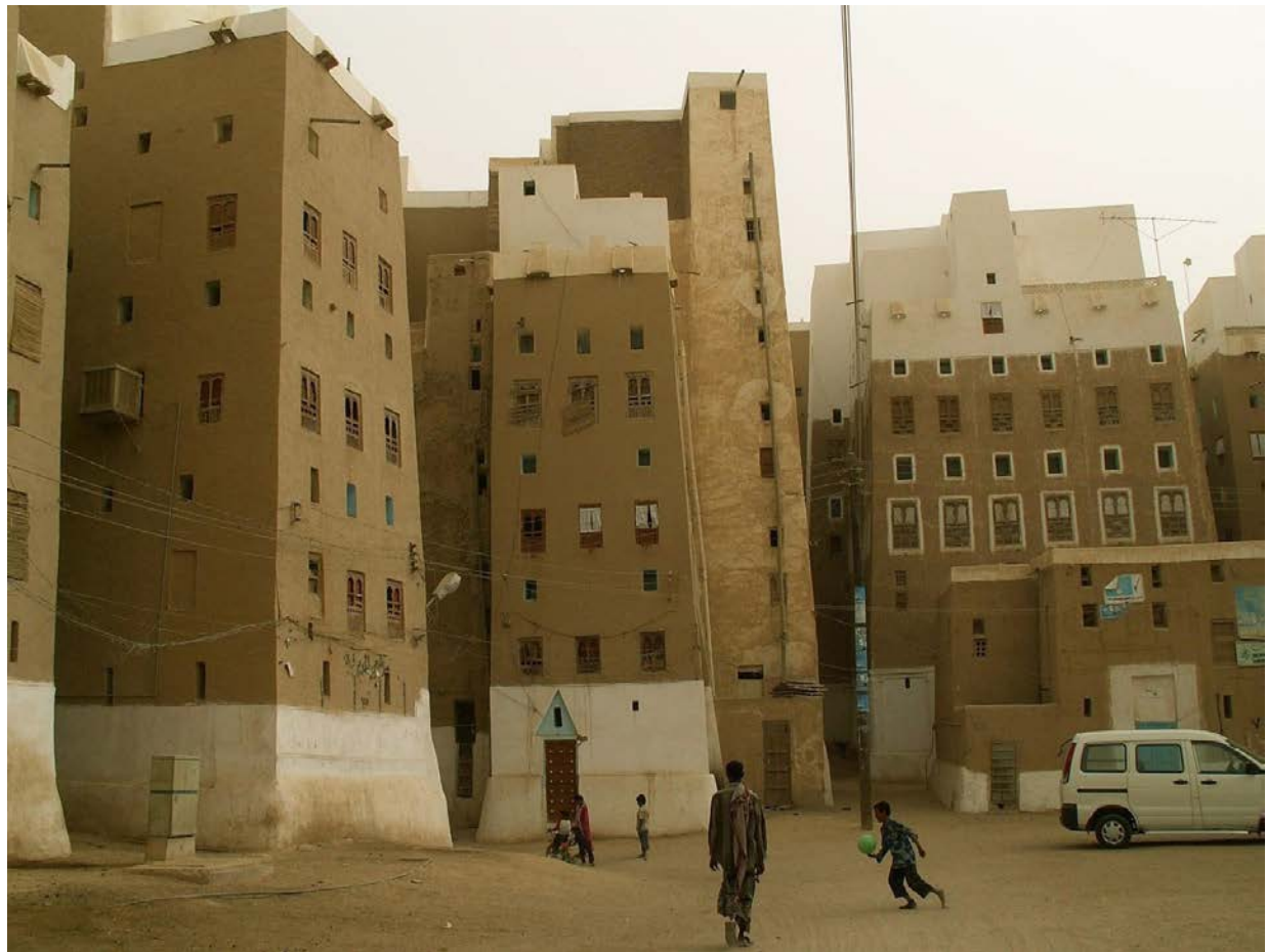
Figure 7. View of children playing in front of tower houses in Shibam
