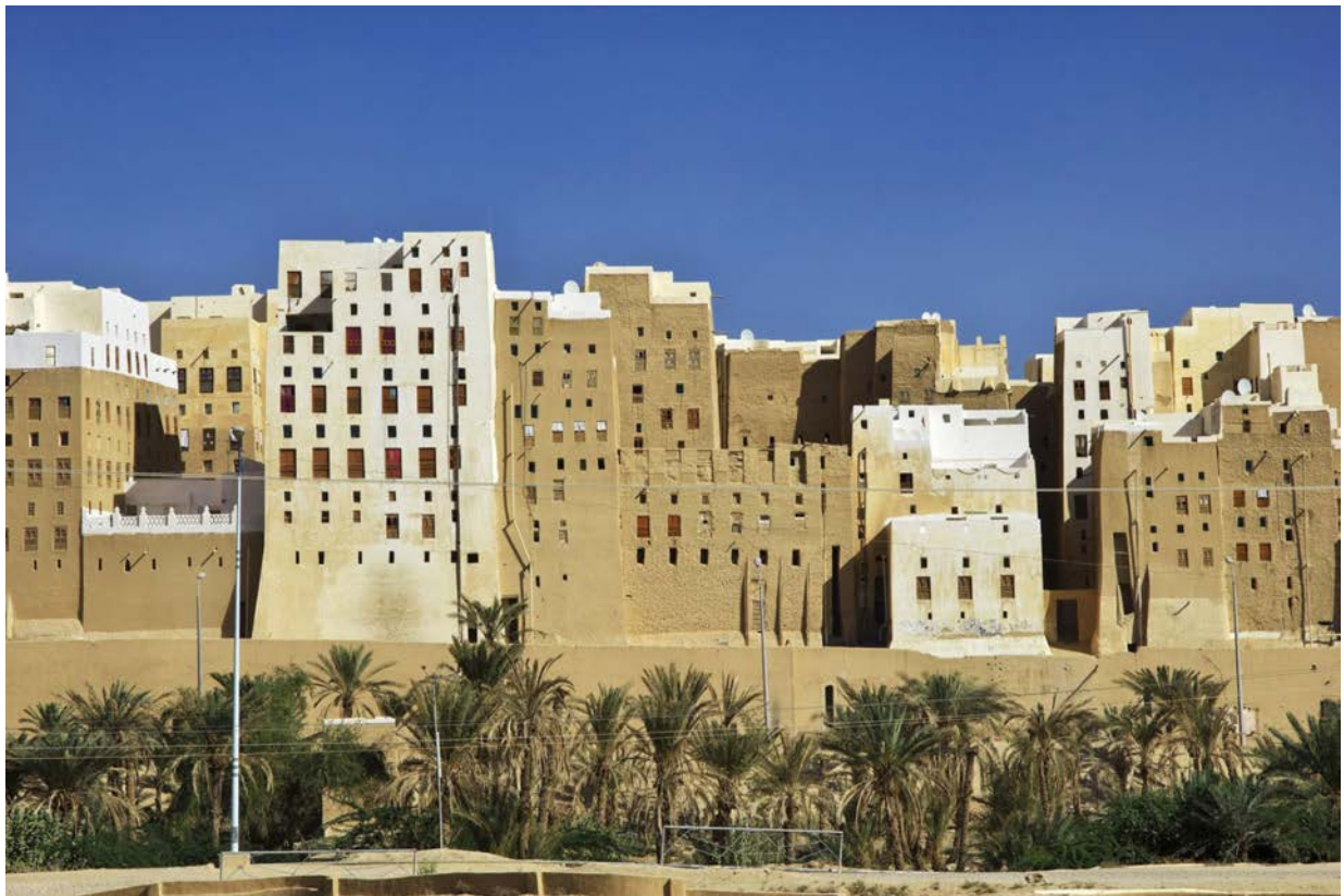
Figure 5. Front view of a row of buildings in Shibam
