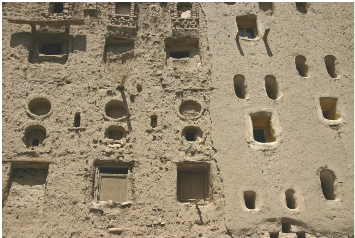
Figure 10. Earthen wall construction and surface maintenance on a tower house in Shibam
