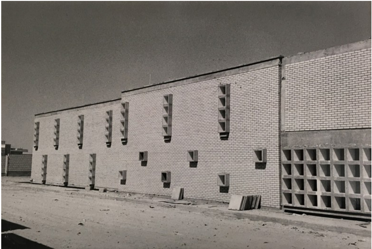
Figure 13. Exterior facade, Alfred Roth school, Kuwait, showing brick construction, hooded ventilation outlets, and minimal glazing. Source: Tosland, Ben A., 'New Research: Alfred Roth's Criticism and Answer to Early Schools in Kuwait,' Transnational Architecture Group, 19 December 2017. transnationalarchitecture.group .
