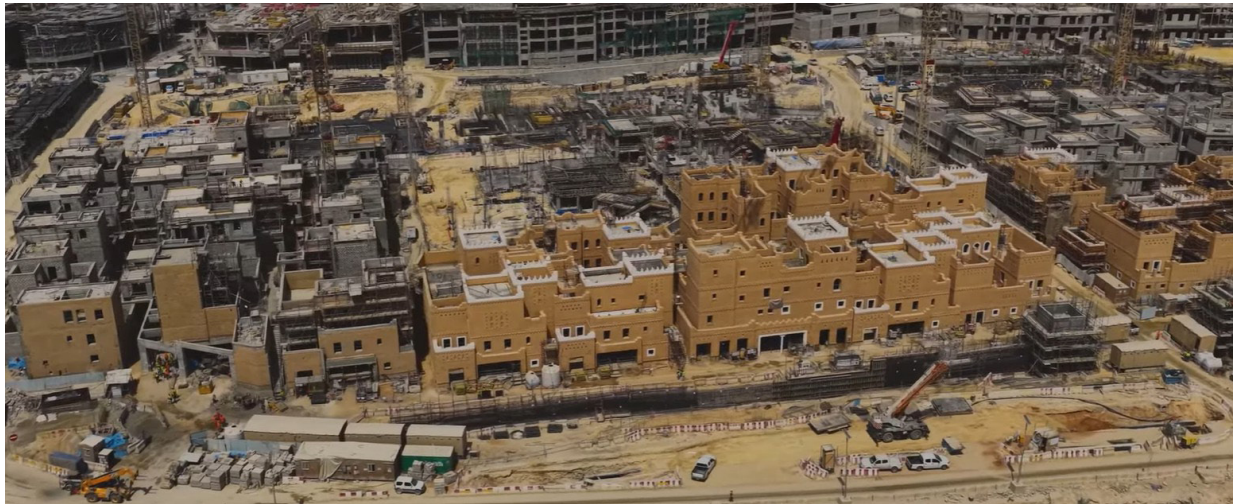
Fig.14 - Ritz-Carlton Residence Construction in Diriyah, showing the use of reinforced concrete.
