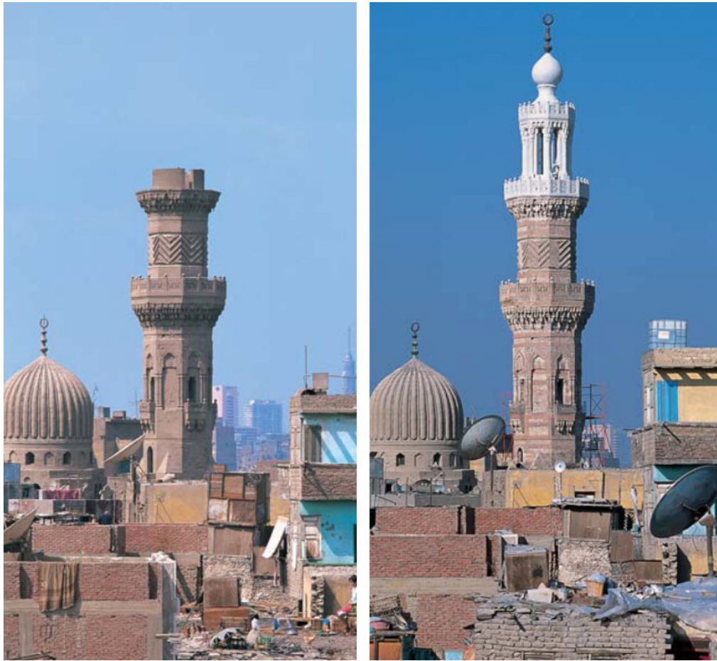
Fig. 6 - Before and after the reconstruction of the Um al-Sultan Shaaban Mosque minaret. From the Aga Khan Trust for Culture. Cairo: Urban Regeneration in the Darb Al-Ahmar District—A Framework for Investment . Geneva: Aga Khan Trust for Culture, 2005, 42.
