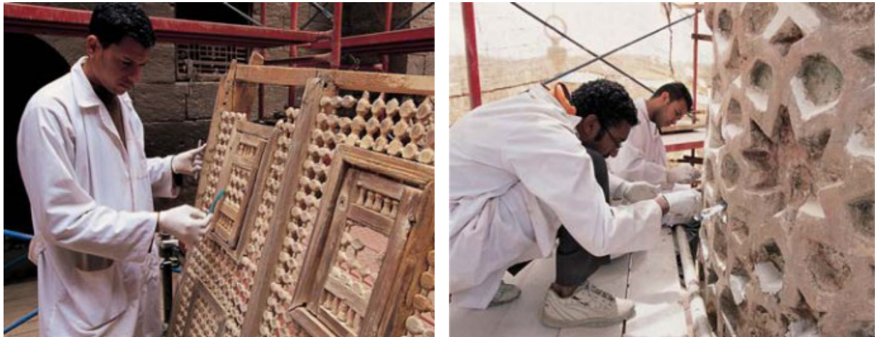
Fig. 7 - (Left) Restoration of a Khayer Bek mashrabiyya screen in a wood conservation workshop. (Right) “Painstaking” restoration of the decorated shaft of the Khayer Bek minaret.
