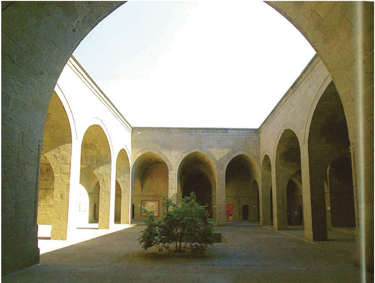
Figure 01. The Courtyard of the Healing Center. The small corridor near the entrance leads to the Mental Asylum. Abdullah Kılıç, Kayseri Gevher Nesibe Şifahanesi ve Tıp Medresesi 1206 = Kayseri Gevher Nesibe Hospital and Medical Academy 1206 (Medical Park Hastanesinin kültür hizmetidir, 2007). 34.
