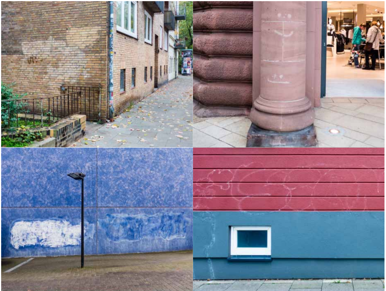
Fig. 8 - Regardless of the substrate, chemical-based graffiti removal often produces poor results. Hamburg, Germany. 2016. Photos by D. Huntington.
