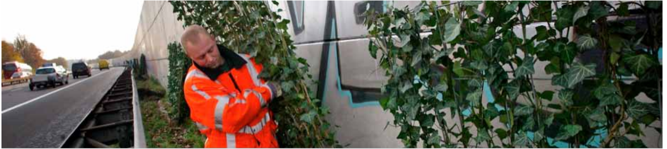
Fig. 14 - Going 'green against graffiti' on retaining walls. Zwolle, Netherlands. 2016. Photo by Mobilane.
